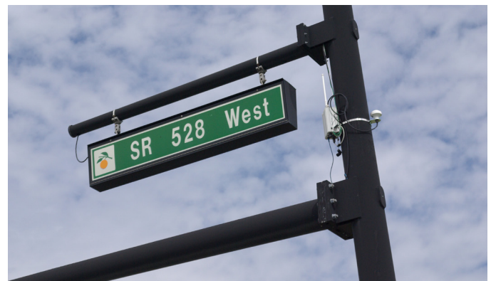
5. Roadside Equipment (RSE) at International Drive and SR 528
